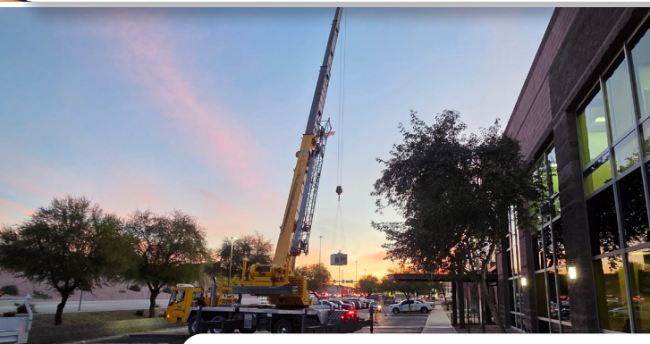
Crane installing new AC units
